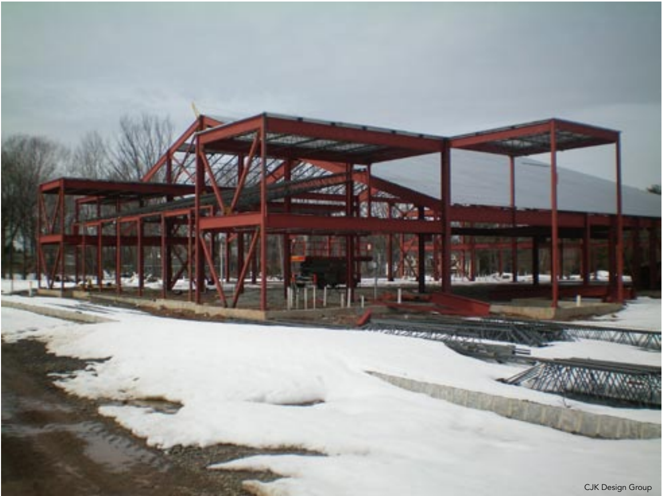
▲ Erected structural framing for the gymnasium building.
