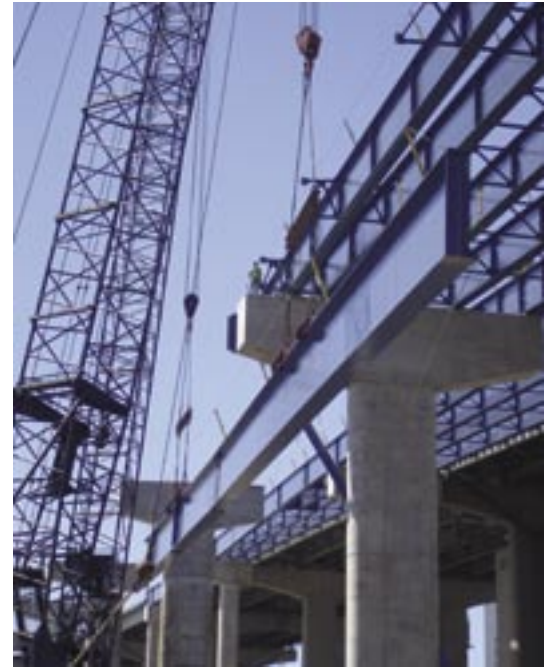
Steel plate girders being erected. Photo by Robert Wazniak, WisDOT.
