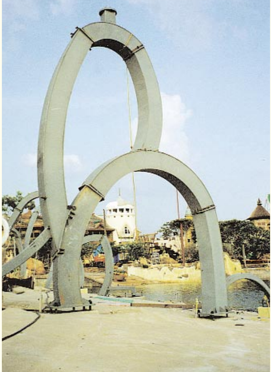
Photos courtesy Walter P. Moore, Houston, TX.
