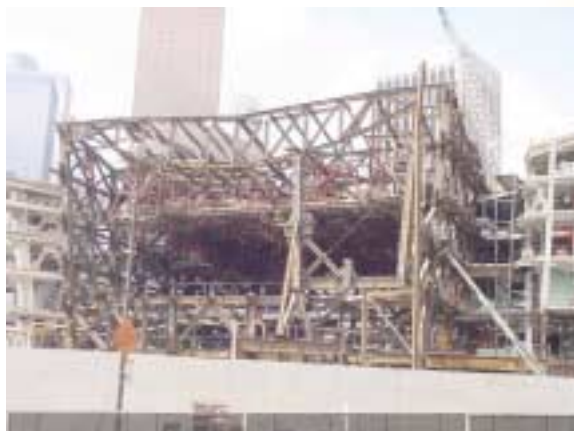
Walt Disney Concert Hall under construction.
