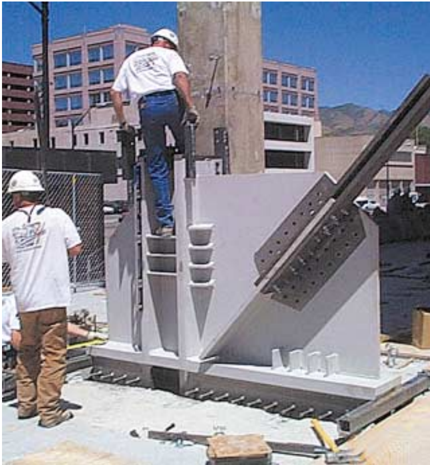
Fig. 4.b. Brace connection assembly ready for installation at grid line Q'-2'.
