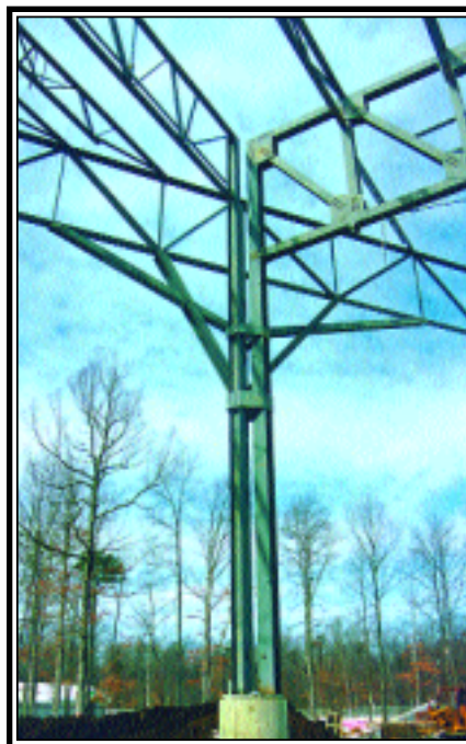
The use of large trusses supported on giant “tree” columns located in aisles resulted in wonderful sightlines for visitors to the Nissan Pavilion near Manassas, VA. (Photography by Hoachlander Photography Associates)
