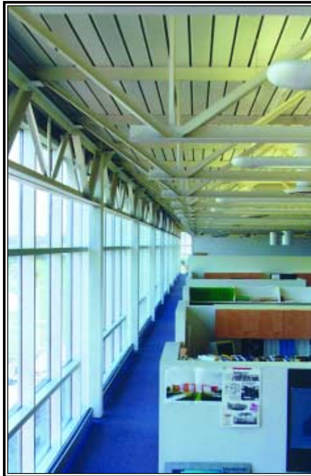
Exposed joists and tubular columns helped create an open feeling for Flad & Associates' new headquarters in Madison, WI.
